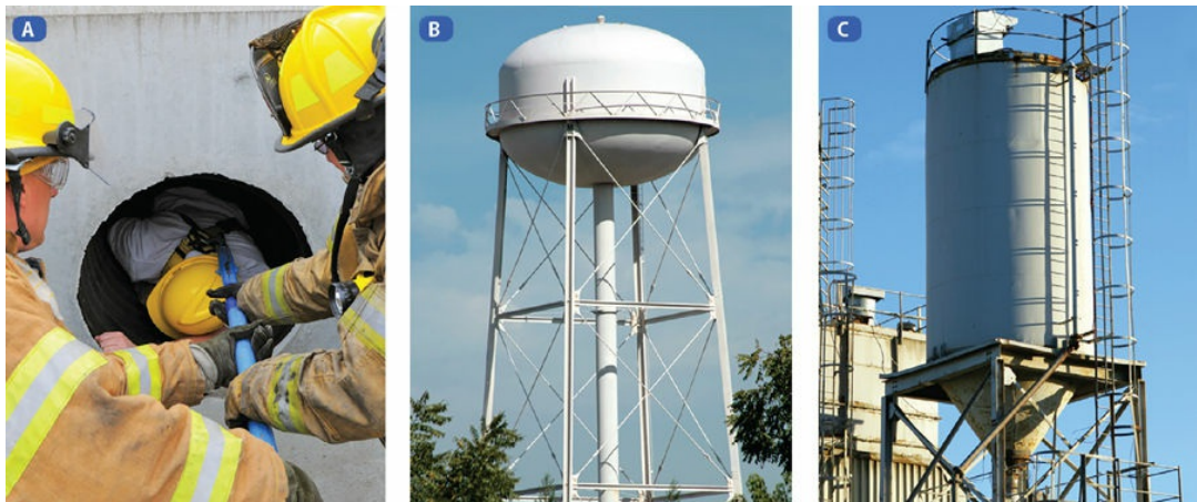
Figure 20-17 Confined spaces may have insufficient oxygen to support life without the use of a self-contained breathing apparatus.
